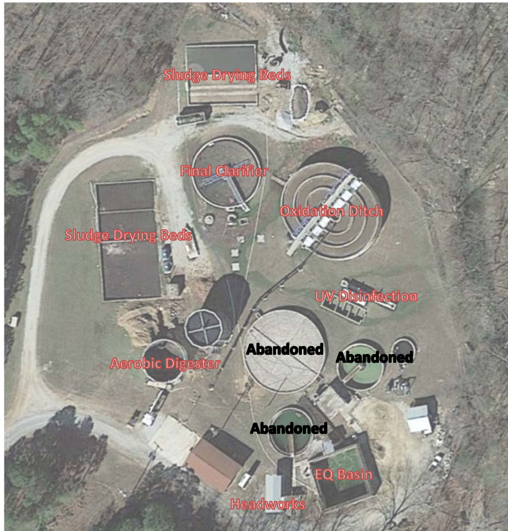
Image 3.1 - Mt. View WWTP Aerial Photo
